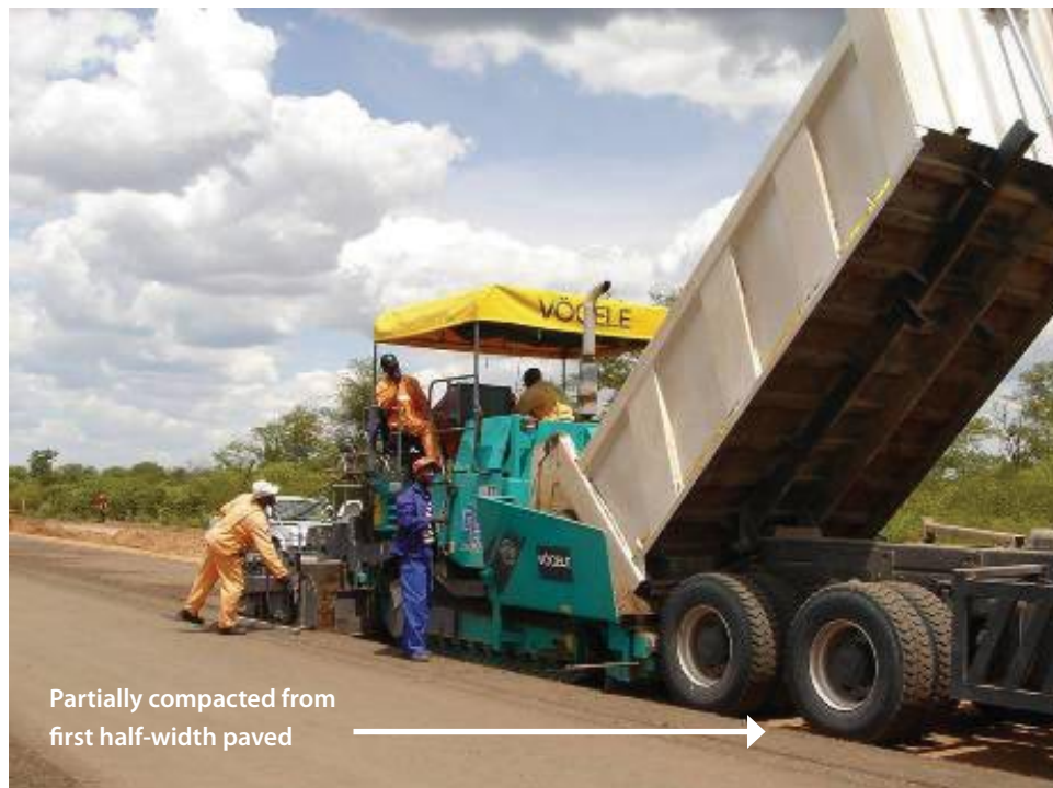
Figure 6.10 Longitudinal Joint Treatment
