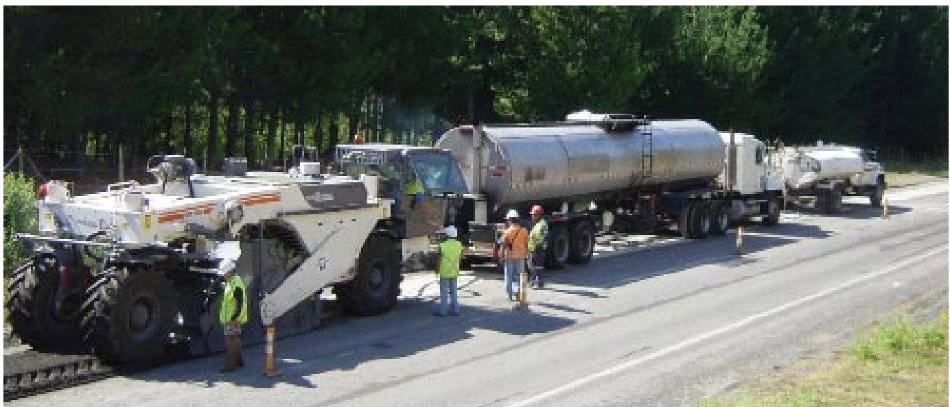
Figure 6.7 Typical Recycling Train for Bitumen Treatment
