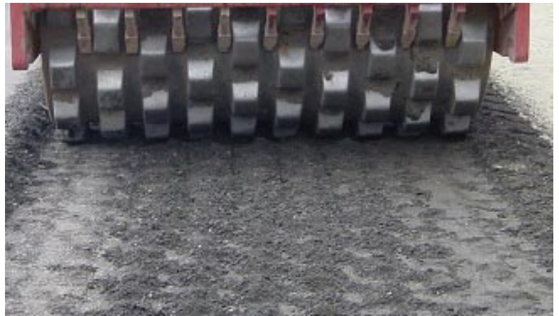
Padfoot roller “walking out” of compacted material leaving “pockmarks”
