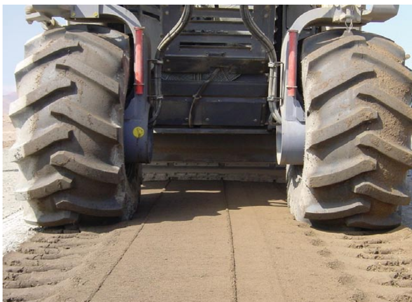
Figure 6.8 Material Compacted by the Rear Wheels of the Recycler
