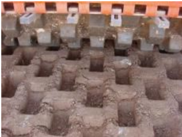
Deep imprints of padfoot roller (Initial stage of compaction)
