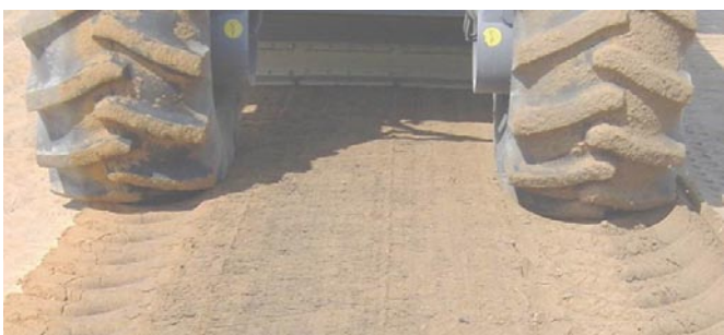
Minimal material sticking to the wheels of the recycler
