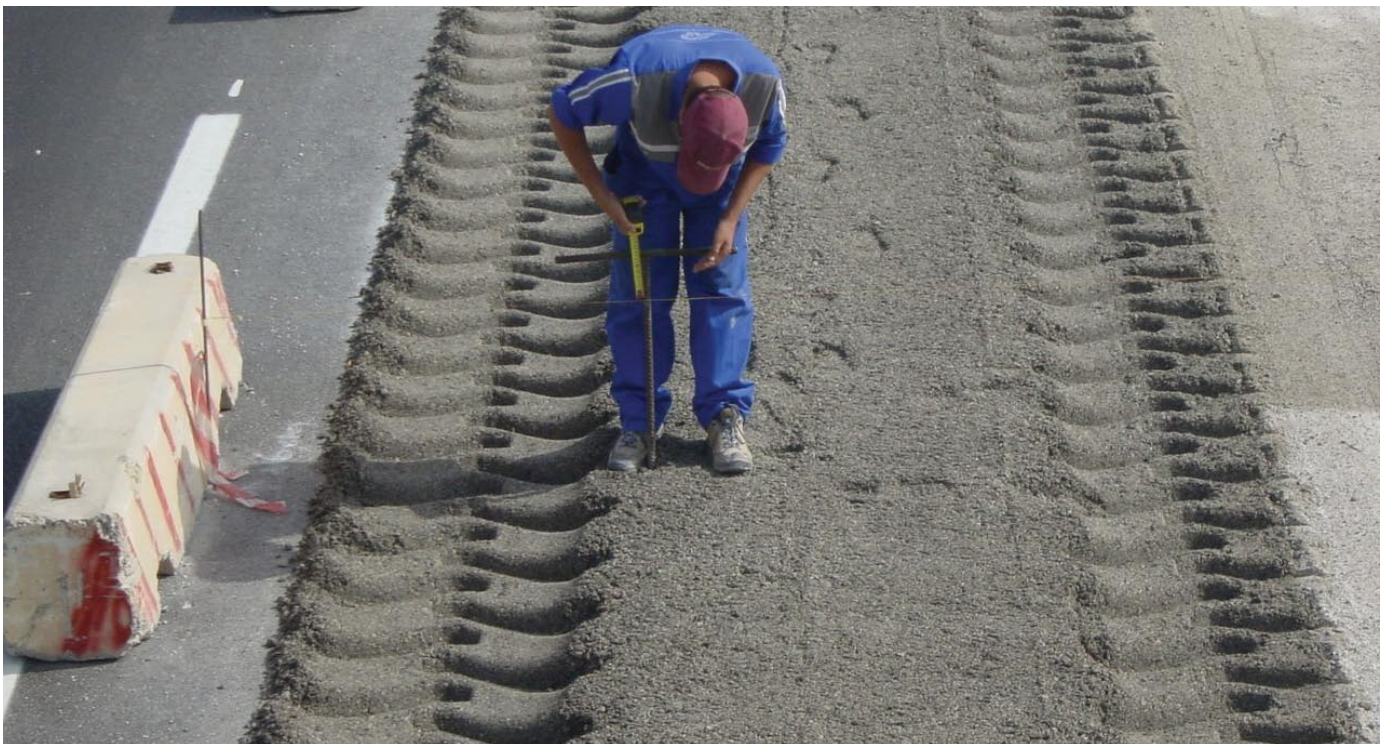
Figure D.1. Where check measurements are taken on the side face of the cut, cognisance must be taken of the increase in surface elevations of recycled material caused by bulking.
