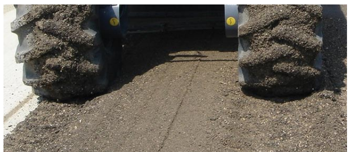
Material sticking to the wheels of the recycler
